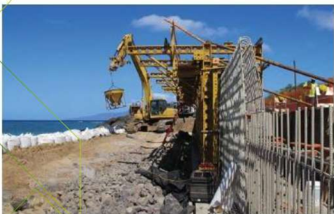
Fig. 3.2f—Construction of seawall with GFRP bars.
